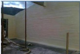
This rigid polyurethane foam has a high potency thermal isolation and completely eliminates the thermal spots.
