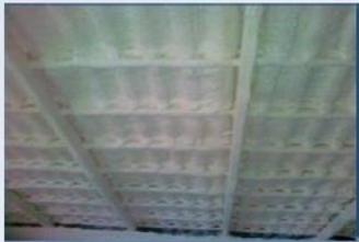
Polyurethane is a solid product, with a foam texture and an appearance between cork and polystyrene. It results from the chemical reaction which is produced almost instantaneously between two liquid chemical compounds. One of these chemical compounds is a reaction activator (known as MDI-isocyanate) and the other is a chemical compound known as polyol.
